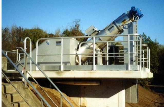
Figure 33 – Membrane Screen RoMEM with enclosure and frost protection package
