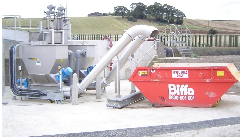
Figure 38 – Screenings washer/compactor with laundry feed - Clayton West, UK
