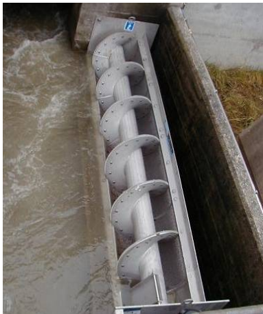
Figure 26 – Stormwater screen RoK1 installed at overflow weir
