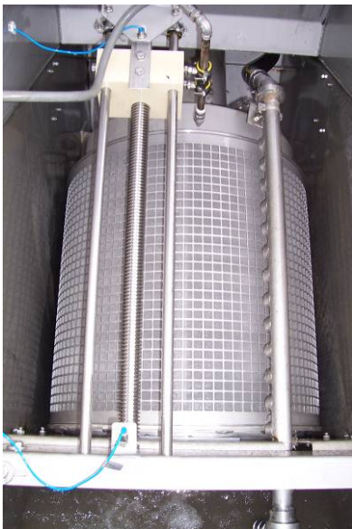
Figure 34 – Membrane Screen RoMEM with 0.5mm woven mesh
